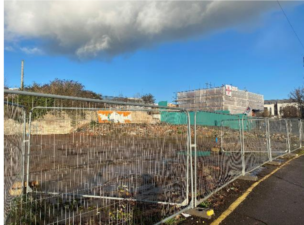
View of site looking eastwards towards block of flats and old railway building
